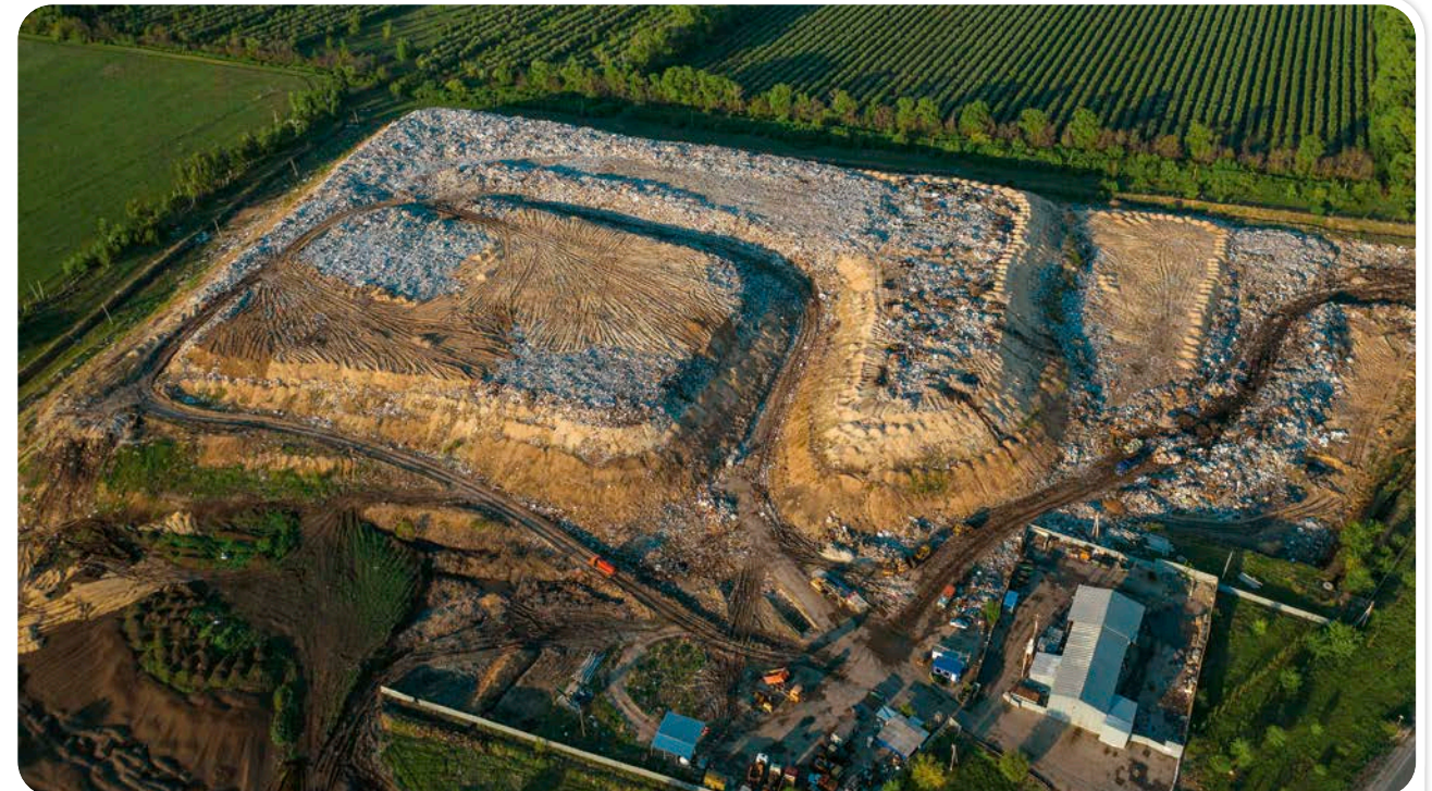
Aerial image of an urban landfill
